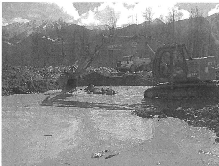
PVDD carrying out sediment removal to restore channel capacity.
