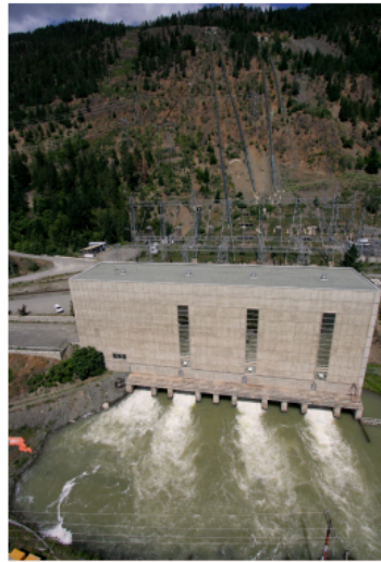
Bridge River Generating Station 1
