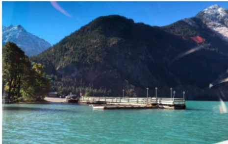
Completed dock work includes new lighting.
