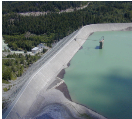
La Joie Dam
