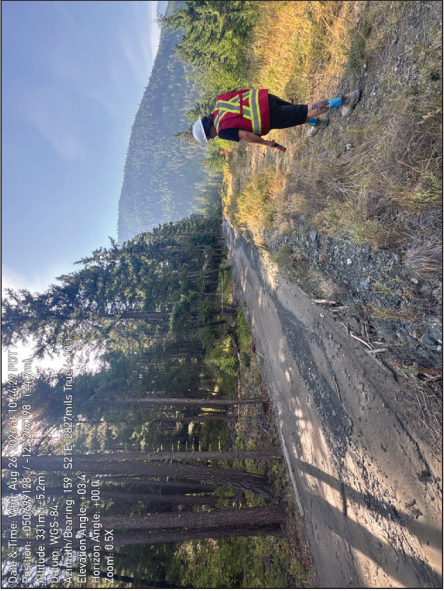
Photo 5. On eastern berm looking south at debris conveyed to the north by the perimeter ditch.
