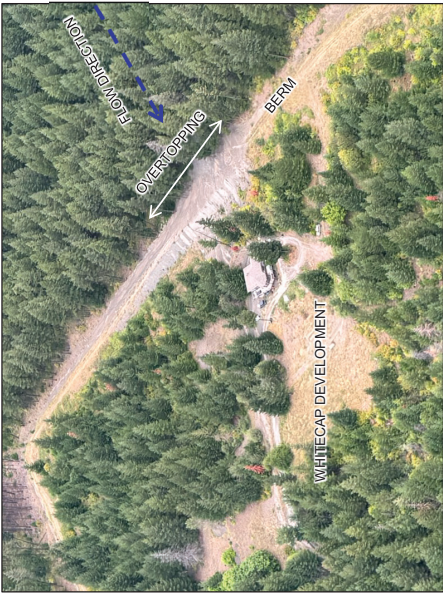
Photo 2. Berm overtopping location from debris flow on Pete's Creek.
