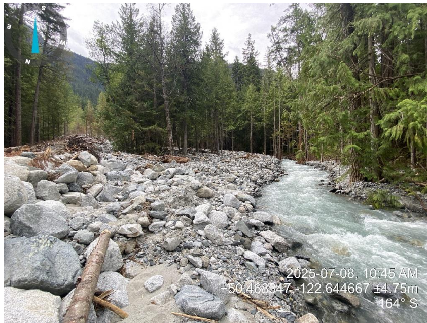
Figure 3-16 Looking upstream at re-channelized flow along the 2024 emergency response channel alignment and deposited sediment and large woody debris along the right riprap embankment
