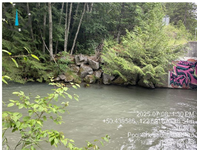
Figure 3-32 Estimated 250-kg MOTT class riprap along upstream left bank of wingwall
