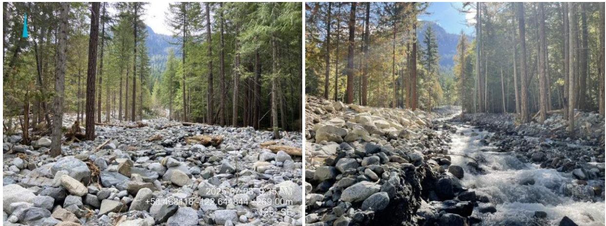
Figure 3-14 Looking upstream where channel gradient flattens and 2025 outburst sediment has filled the 2024 emergency response channel (left image 2025, right image 2024)
