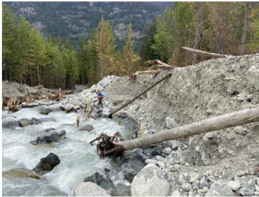
Figure 3-12 Looking downstream towards failed riprap and vertical face of eroded embankment
