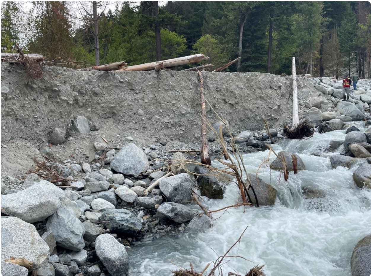
Figure 2-5. Riprap Failure & Embankment Retreat – Looking Upstream (June 8, 2025)
