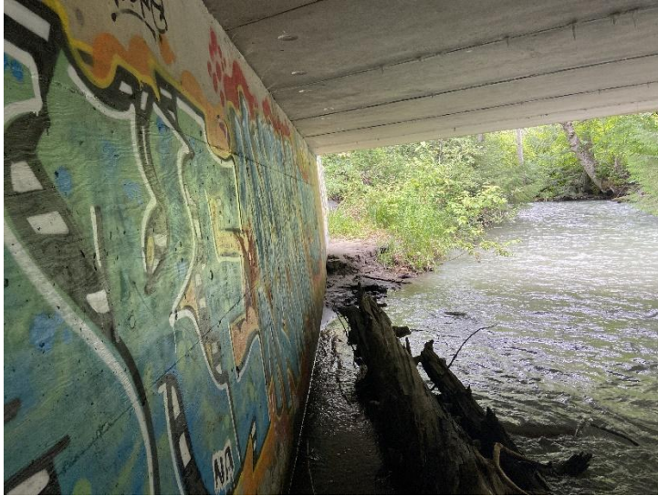
Figure 3-33 Evidence of sediment deposition along upstream right bank of Pemberton Portage Road Bridge
