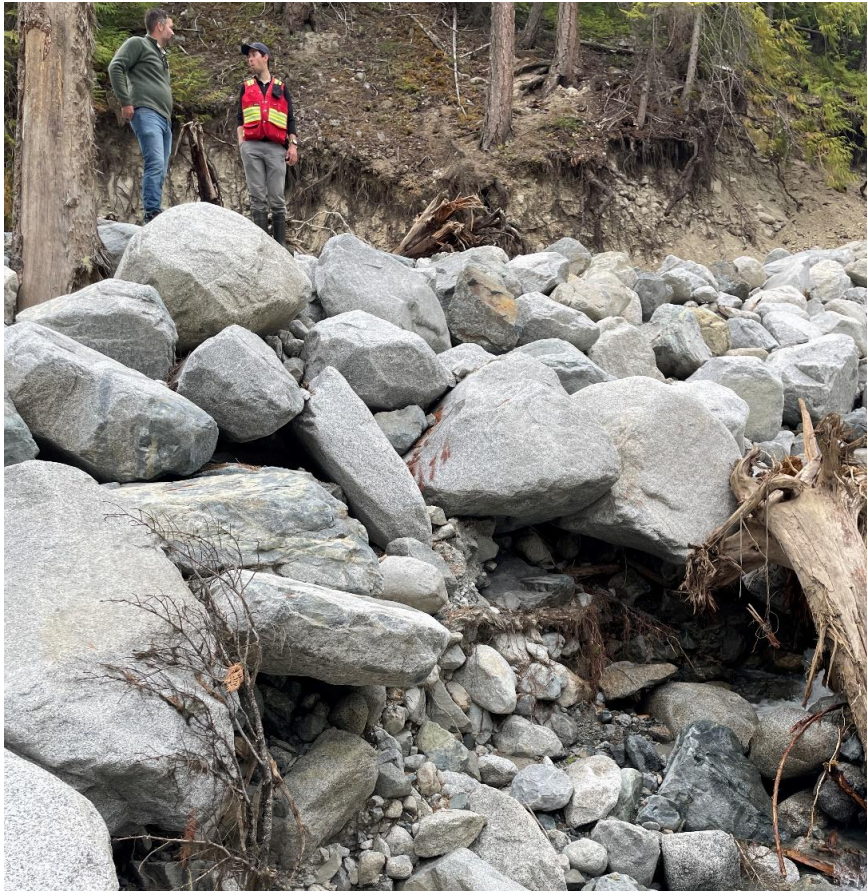
Figure 3-10 Localised areas where scour and incising of channel has undermined right bank riprap
