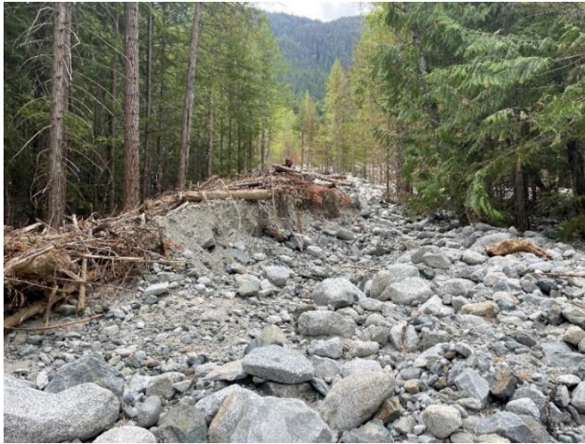
Figure 3-18 Failed portion of right embankment and riprap
