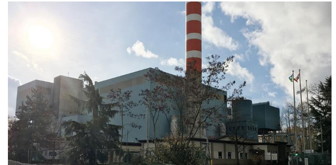
Metro Vancouver WTE Facility
