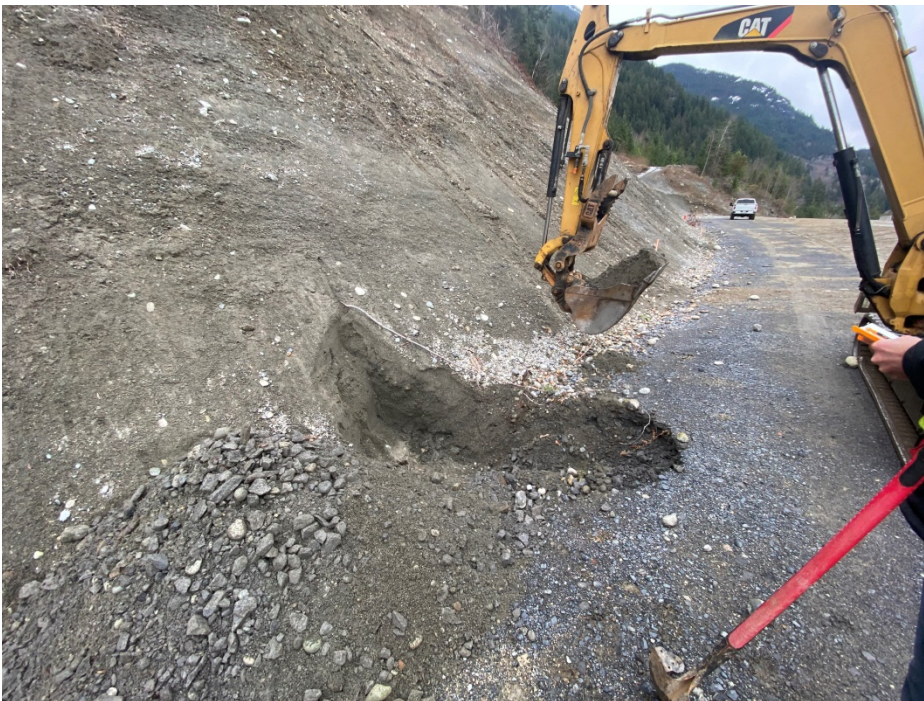
Figure 2 - Testhole 2 looking south (north end Area 2)
