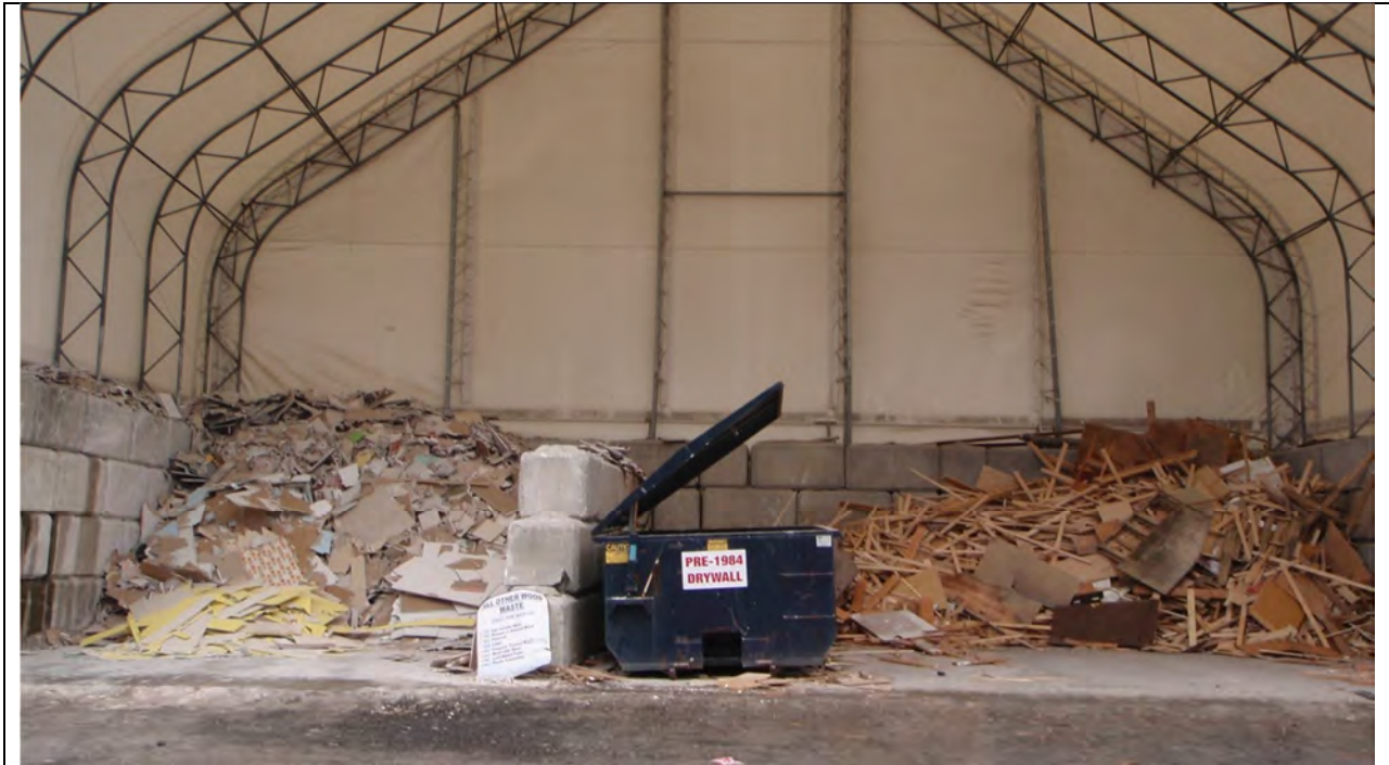
Photo 3 – Drywall and Wood Waste Pile
