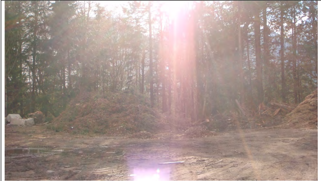
Photo 2 – Yard Waste Pile
