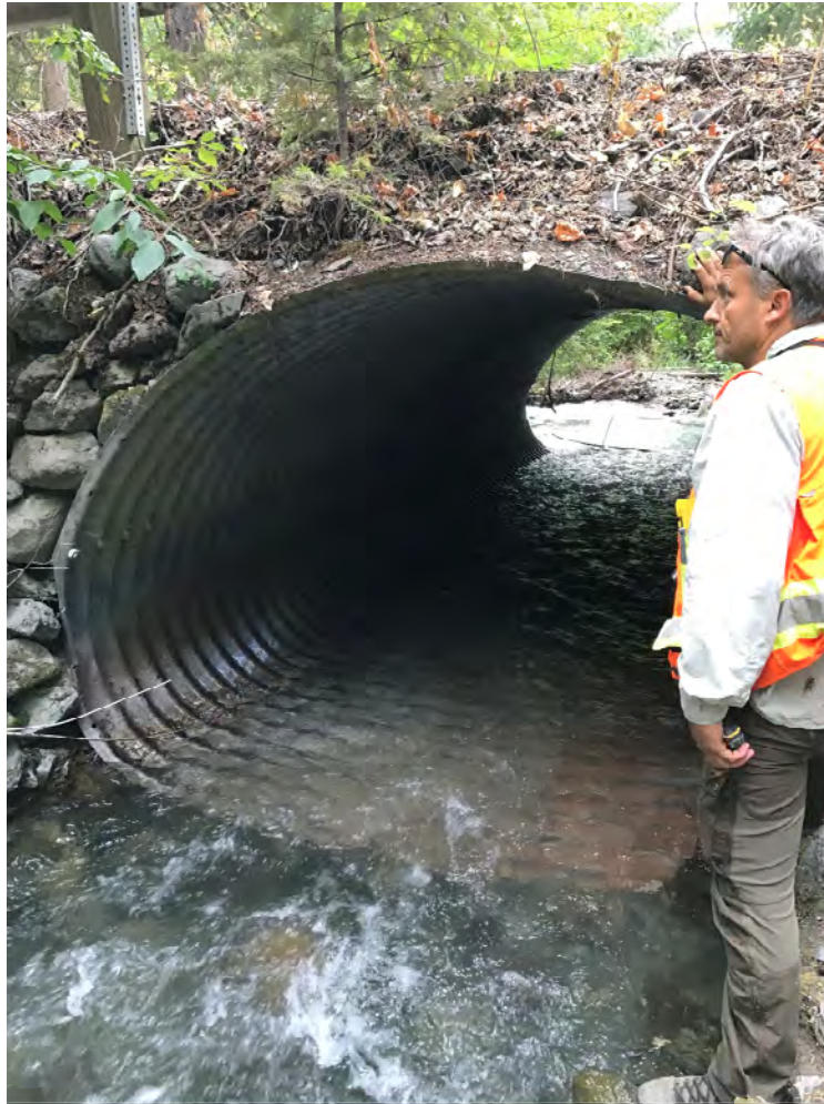
Figure 2-12. Downstream view of corrugated steel culvert underneath Spider Creek Road at Spider Creek. Photo: BGC September 13, 2017.
