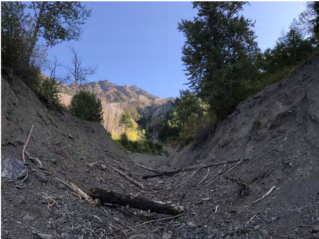
Figure 2-7. Bear Creek channel near fan apex. The channel is incised about 10 m and has a channel gradient of 48%. Bear Mountain in the background. Photo: BGC September 12, 2017.
