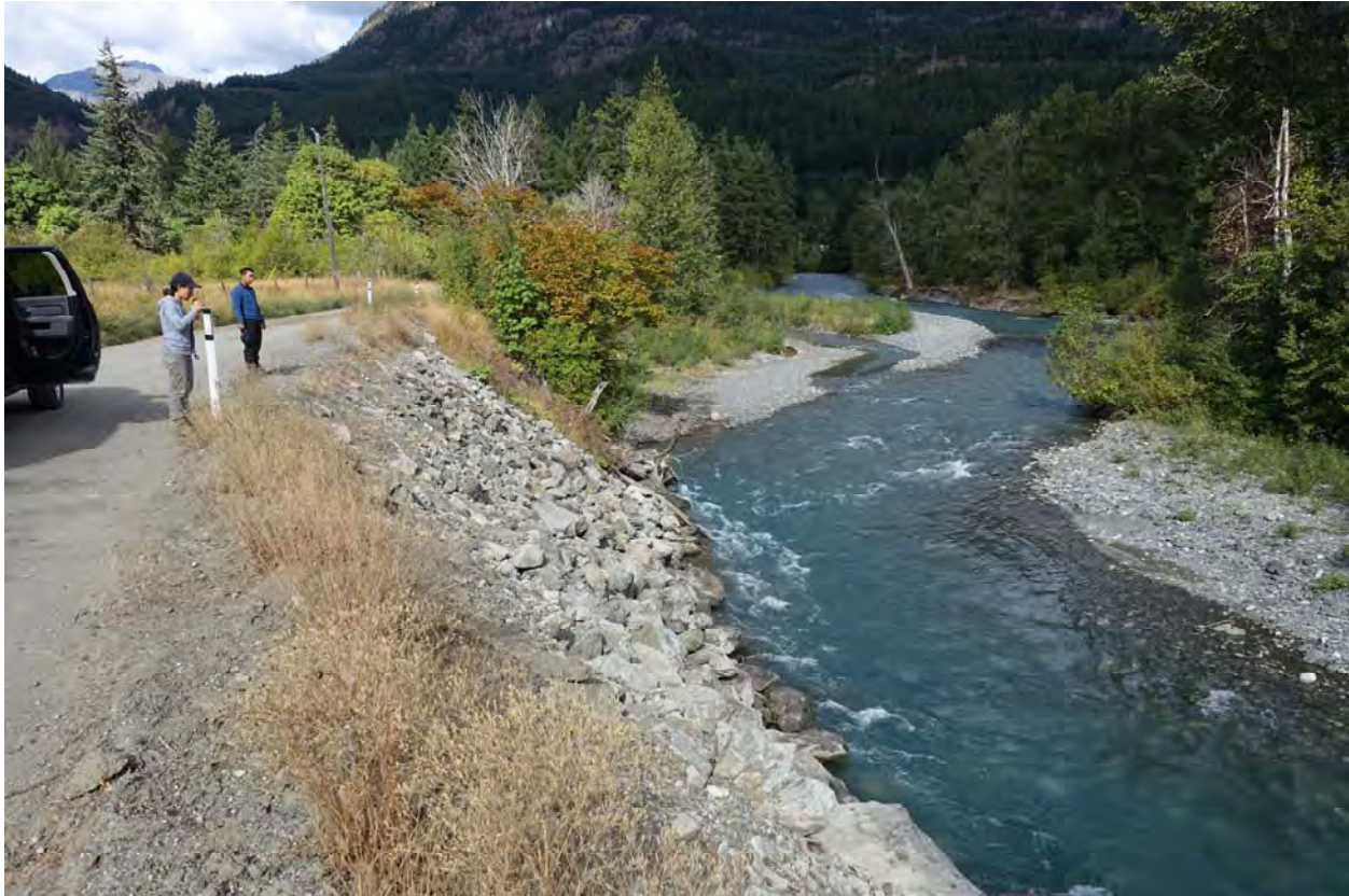
Figure 7-3. Bank erosion at Spider Creek Road. Photo by BGC dated September 13, 2017.
