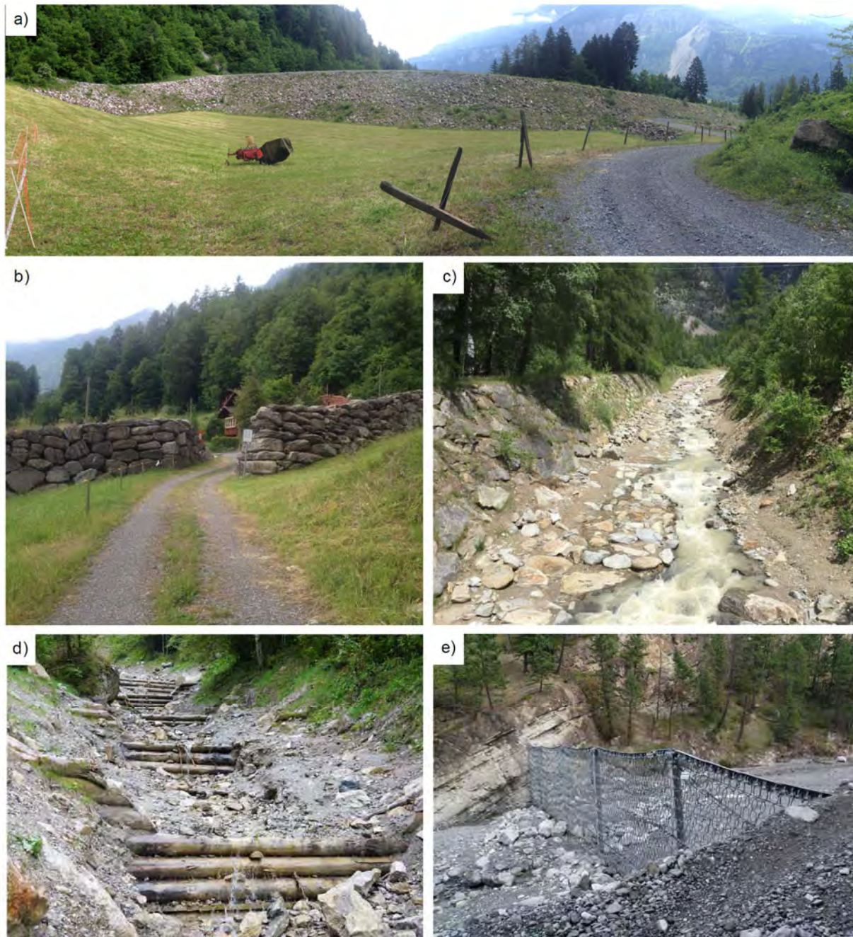
Figure 3-8. Examples of debris-flow mitigation structures: (a) an earth-fill retention berm on Glyssibach, Brienz, Switzerland; (b) a stone diversion berm, Trachtbach, Brienz, Switzerland; (c) a conveyance channel with earthfill berms, Rennebach, Austria; (d) log crib check dams, Gesäuse, Austria; and (e) a flexible debris net for debris flood mitigation, Cougar Creek, Canmore, Alberta. Photograph (d) by M. Jakob, other photographs by E. Moase.
