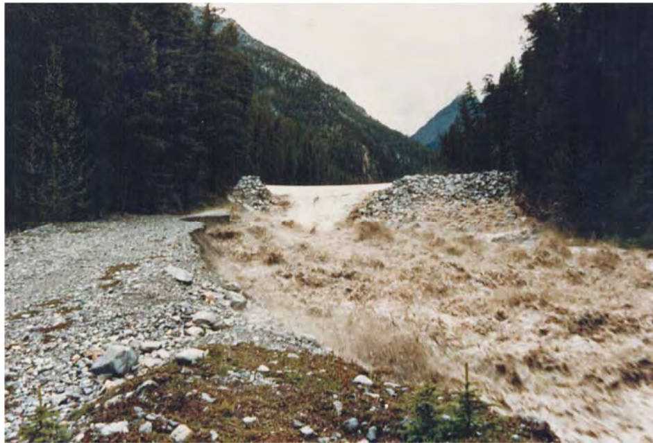
Photograph B-1. Example of the failure of a human-made dam on Cougar Creek shortly after the breach initiated. May 25, 1990 (Alberta Environment 1991).
