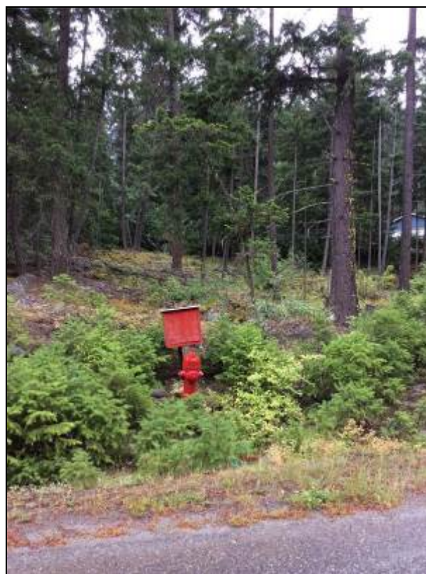
Figure 21. Annually monitor vegetation and remove vegetation encroaching upon critical infrastructure (within 10 m) as needed. Mow all grass and weeds. Remove conifer regeneration (left) and ensure that hydrants and standpipes are easily accessible (right).
