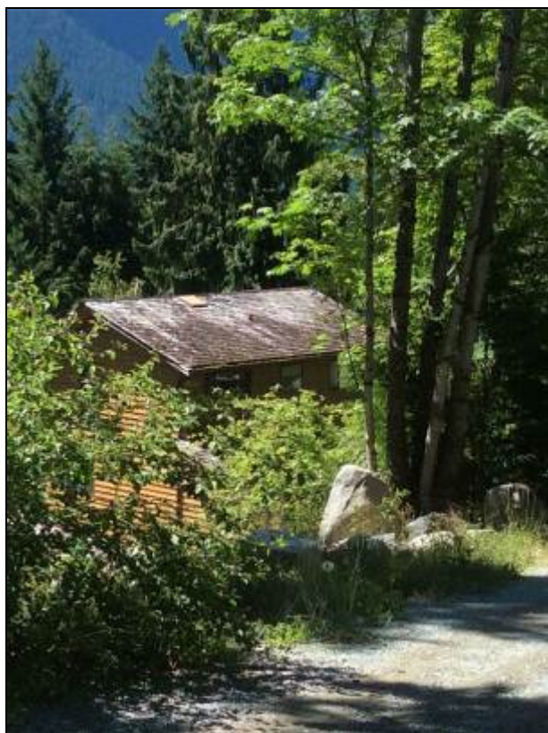
Figure 18. All homes are in a range of FireSmart compliance. Left: residence with unrated shake roofing with accumulations on roof and in gutters. Right: residence with unrated vinyl siding, rated roofing, and FireSmart landscaping, including pruned conifers visible in the far right foreground.
