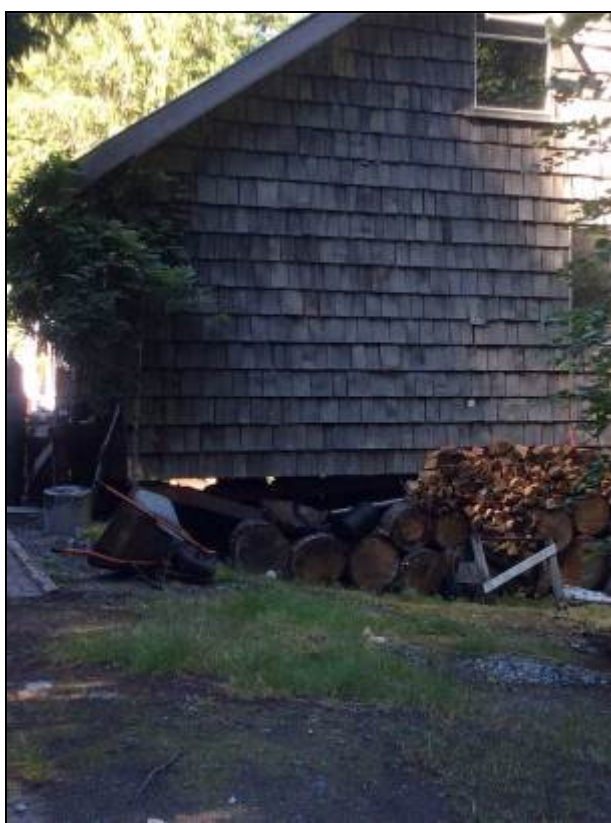
Figure 17. Left: firewood and other combustibles piled adjacent and underneath a residence with cedar shake siding. Right: a preferred alternative, with firewood piled more than 10 m away from the home.
