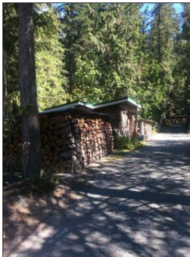
Figure 17. Left: firewood and other combustibles piled adjacent and underneath a residence with cedar shake siding. Right: a preferred alternative, with firewood piled more than 10 m away from the home.
