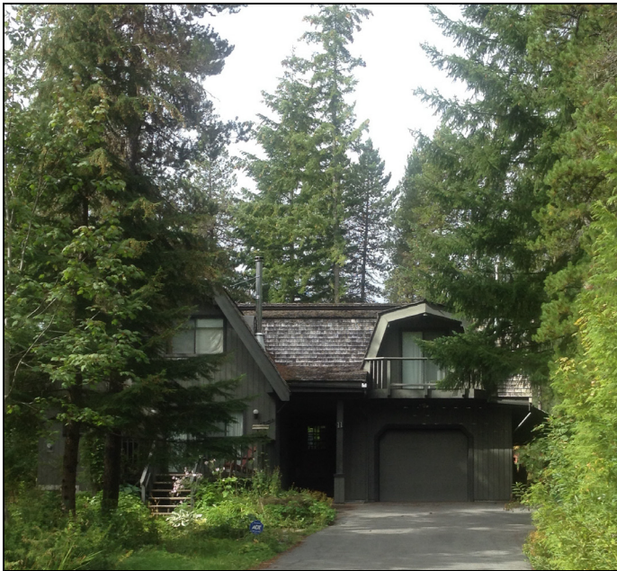
Figure 12. Left: considerable combustible material accumulation on a cedar shake roof. Priority Zone 1 is not FireSmart. Right: a preferred alternative, large timber home with metal roof. It is still recommended to remove all combustible materials from roof (conifer needles). Priority Zone 1 is maintained in a manner closer to FireSmart compliance.
