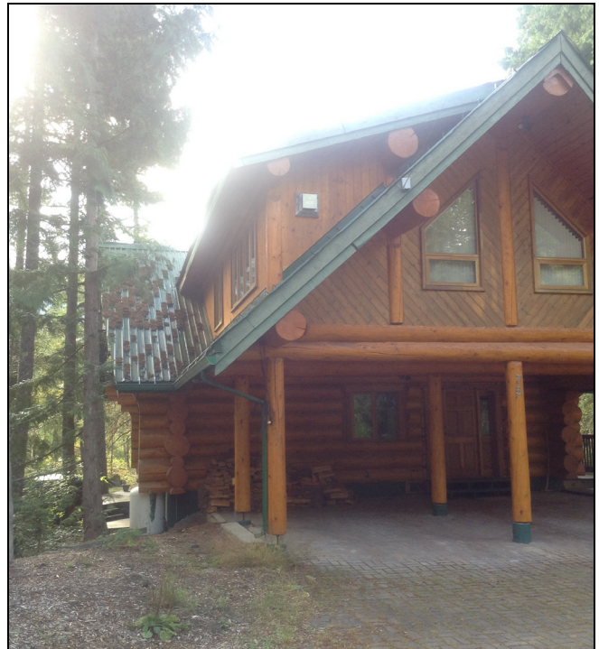
Figure 12. Left: considerable combustible material accumulation on a cedar shake roof. Priority Zone 1 is not FireSmart. Right: a preferred alternative, large timber home with metal roof. It is still recommended to remove all combustible materials from roof (conifer needles). Priority Zone 1 is maintained in a manner closer to FireSmart compliance.
