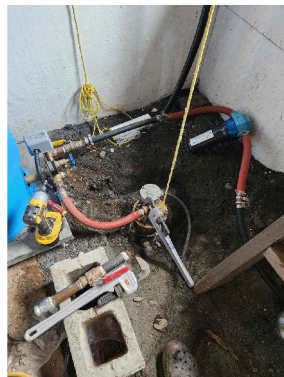
P2: WTN50957 in a concrete pit
