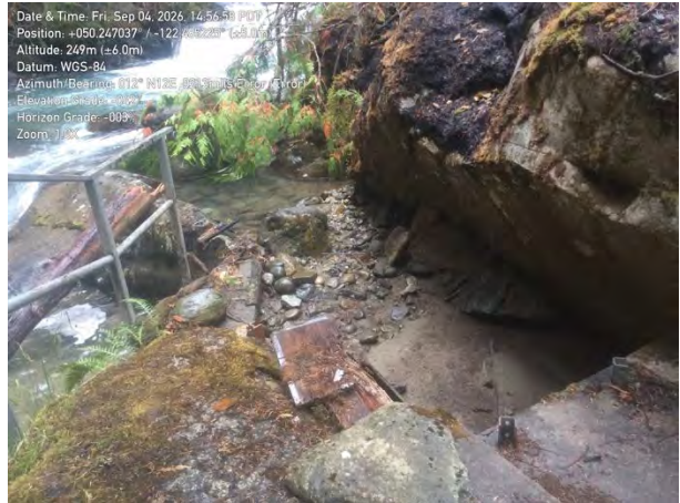
Twin One Intake, abandoned intake flume
