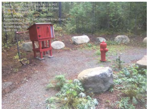
Twin One hydrant station, site 2
