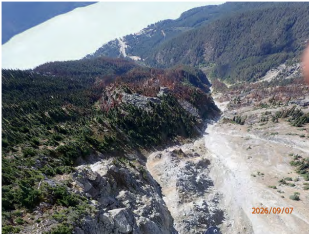
View southwest down Cataline Creek to mitigation works under construction.
