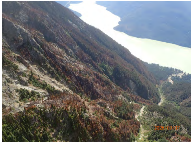
View south down Cataline Creek to mitigation works under construction.
