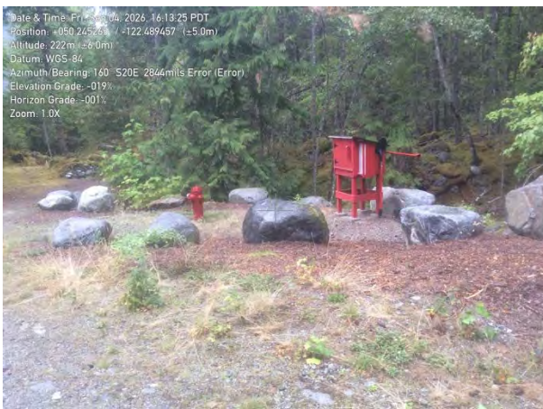
Twin One hydrant station, site 1
