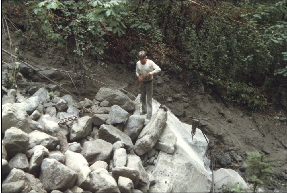
Photograph 1. Breaking of large boulders along the upper portion of Catiline Creek following 1986 debris flow event. Photograph taken by the Hills Family provided by Gary Young dated July 25, 1987.
