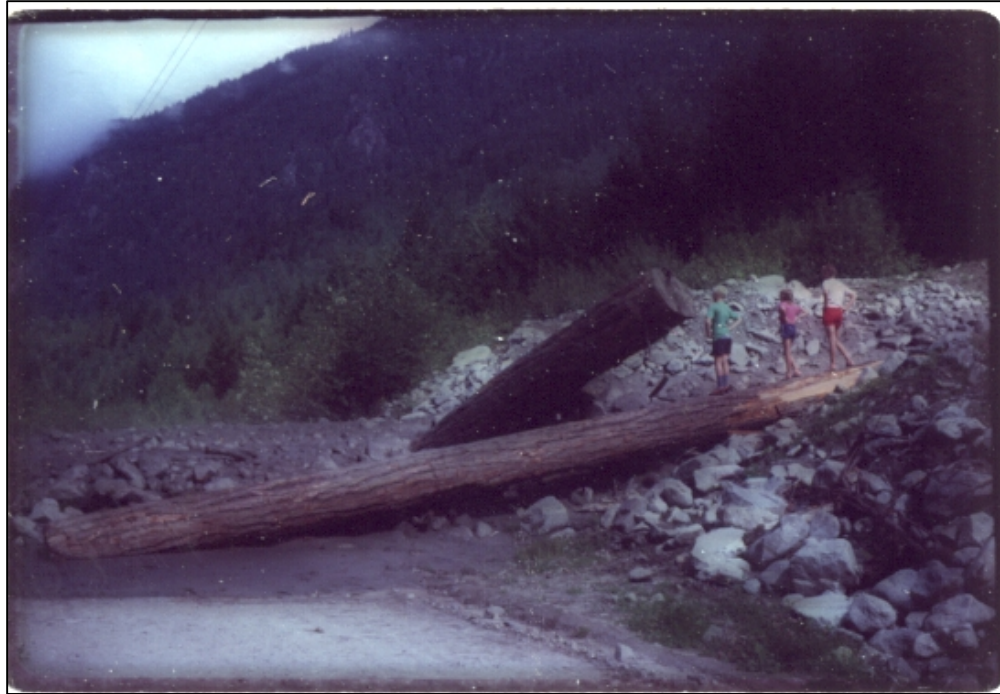
Photograph 5. August 1987 debris flow deposits. Photo provided by the Klassen family. The logs are likely the remains of the check dam shown in Photo 2.
