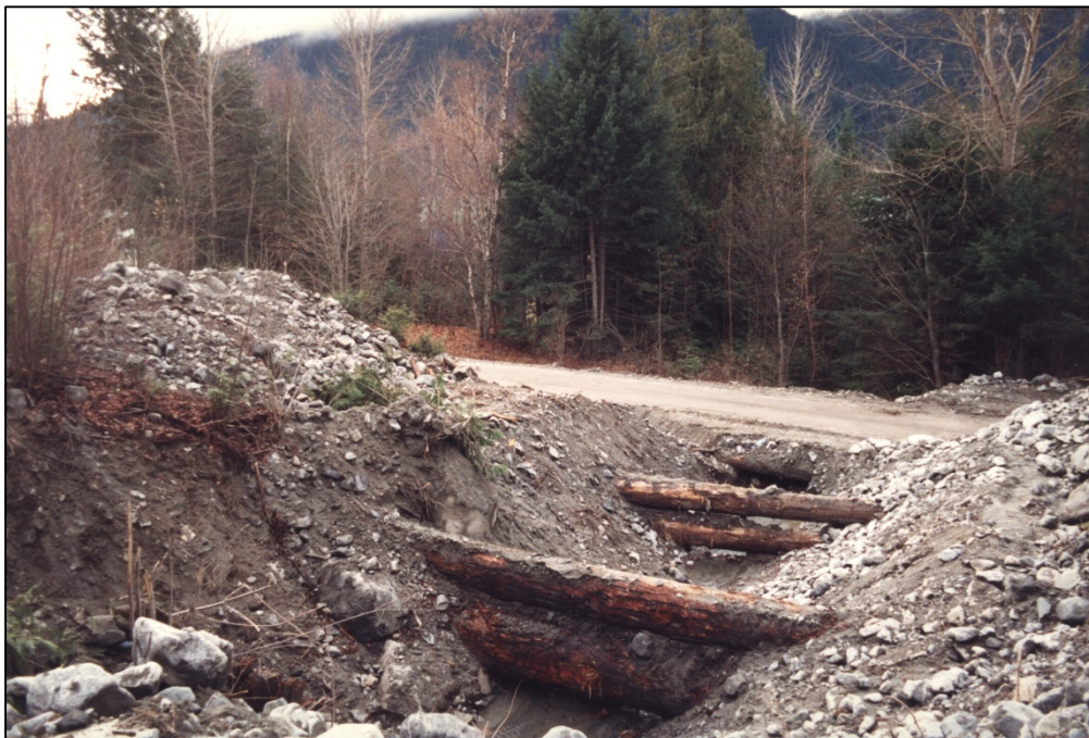
Photograph 2. Looking downstream at debris check dam constructed of wood (no longer existing). Photograph taken by the Hills family, provided by Gary Young dated November 12, 1986.
