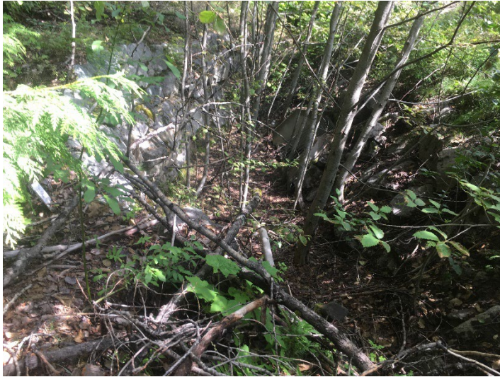
Photo 8. View of Highway 99 culvert at the eastern extent of Drainage 1. July 18, 2019.
