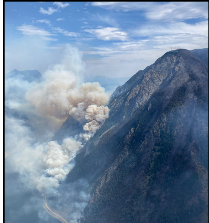
The Casper Creek wildfire looking east over Terzaghi Dam (Aug. 17, 2023)
