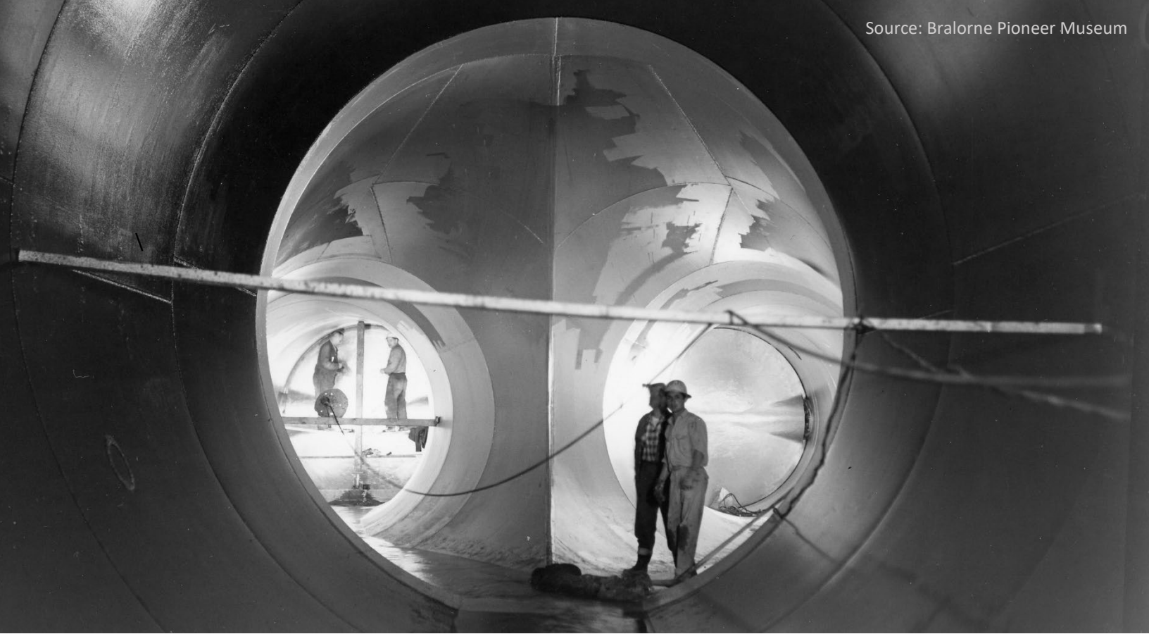
Historical Photo of BC Hydro's Bridge System Penstocks
