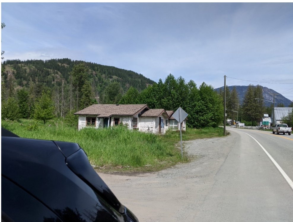
Figure 14 East side of Development site looking north at 2 and 3 of 3 existing structures. Water would flow from north and follow Hwy 99 south across the site
