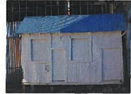
Roots Blower Shed
