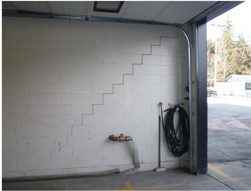
Photo A3 – Settlement Crack in Block Wall
