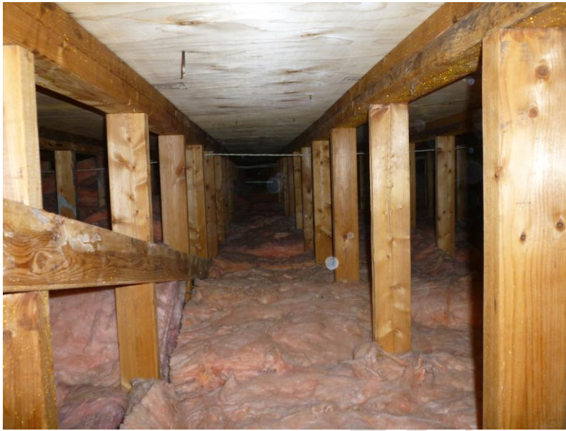
Photo A1 – Pony Walls Supporting Roof Sheathing
