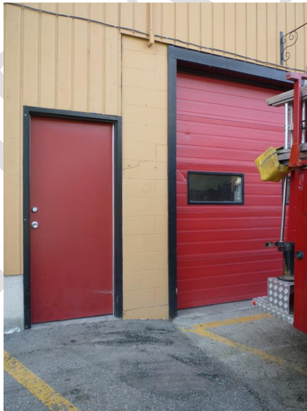
Photo A4 – Diagonal Crack in Block Wall Pier
