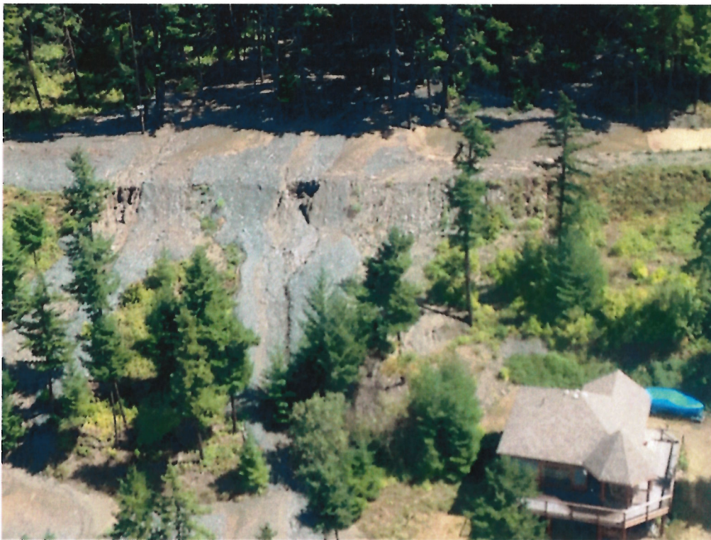
Plate 4: Debris flow deposits overtopping the ditch and berm on Pete's Creek.
