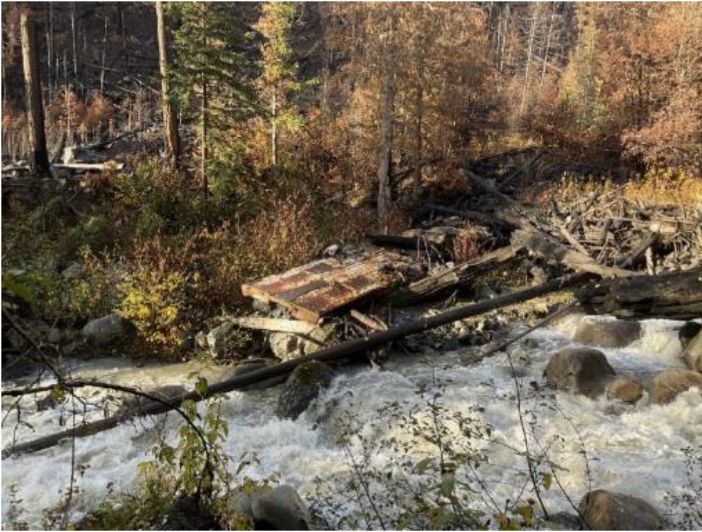
Photo 17 Upper Whitecap Creek bridge that has been previously washed out, looking west.
