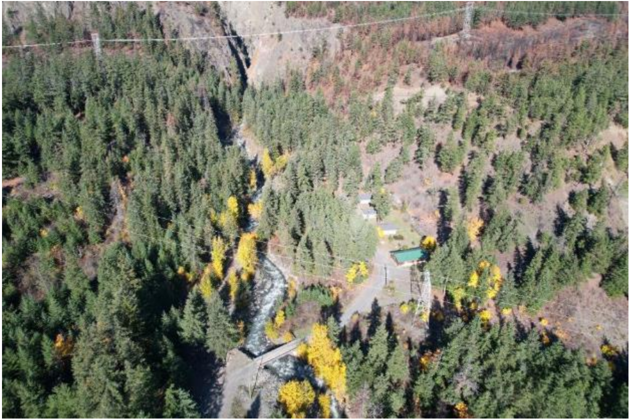
Photo 21 Lower Whitecap Creek with the FSR bridge, cabins and office building.
