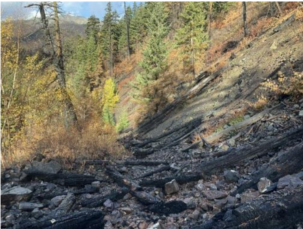
Photo 18 Ravelled scree slope and rockfall deposits on Whitecap FSR, looking north.
