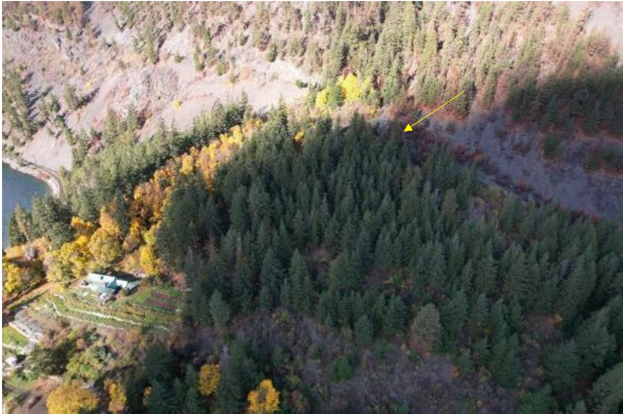
Photo 5 H2 fan below Highline Road. Note BCH transmission line tower near fan apex. Stream is well confined in a large draw adjacent to the structure.
